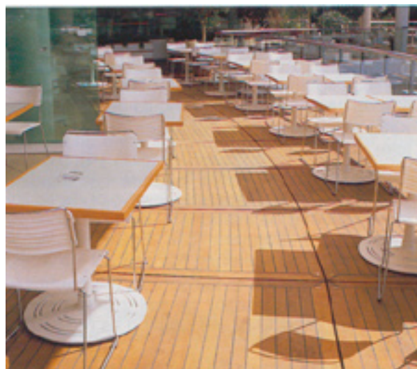
Decking panels fixed over concrete with stainless steel locating bolts – decking boards screw to battens from underside.
