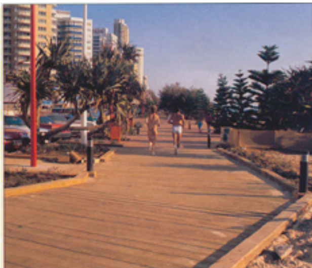
CCA treated softwood decking in exposed beachfront environment.
