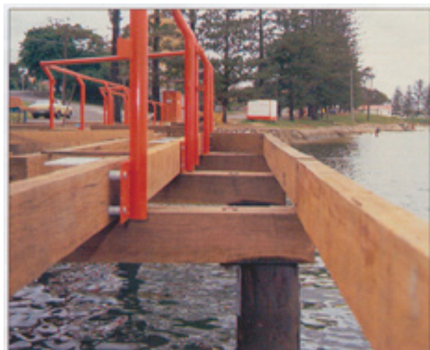
Boardwalk substructure provides fixing base for metal handrails.
