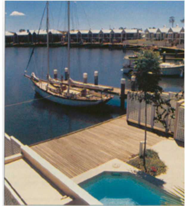
Timber decks provide recreation space and water access in residential development.
