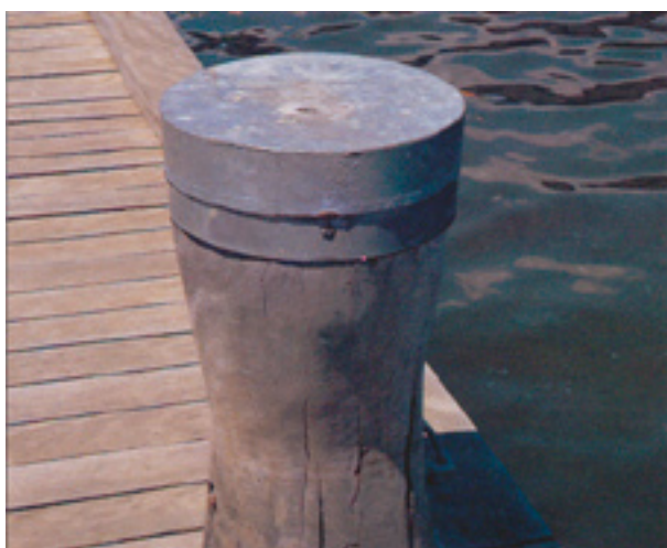
Metal capping provides protection to end-grain of bollard.
