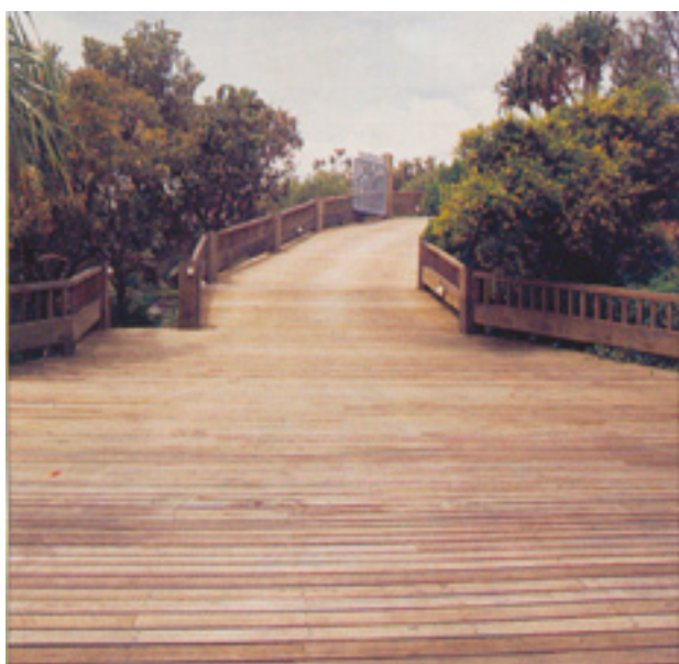
Heavy-duty suspended vehicular access.
