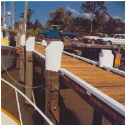
Heavy hardwood decking makes for practical and hard-wearing jetties.
