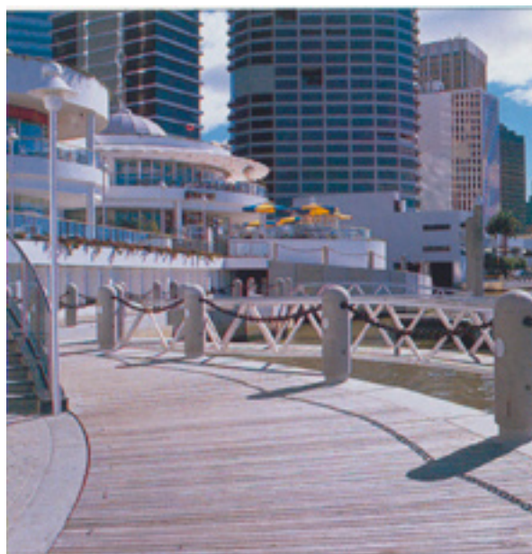
Hardwood decking (120 x 45) set in concrete surrounds, screw fixed from underside – panels located with stainless steel bolts.
