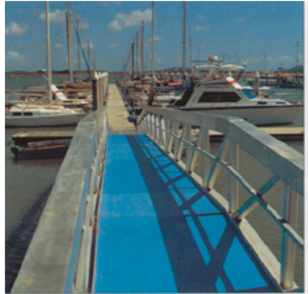
Fibreglass overlaid plywood decking in marina walkway.
