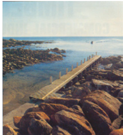
Timber jetty provides access to deep water.
